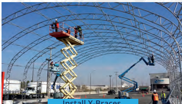
Install X-Braces, Purlins, & Cables
