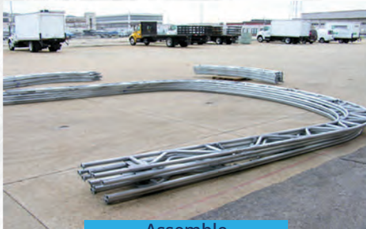
Assemble Truss Frames
